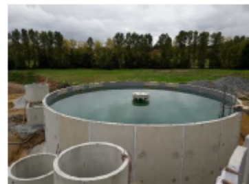
Construction station de St Pardoux Soutiers
